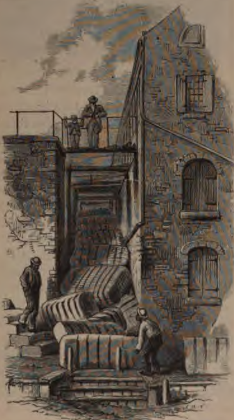
"Looking down from the bluff"—Savannah.
